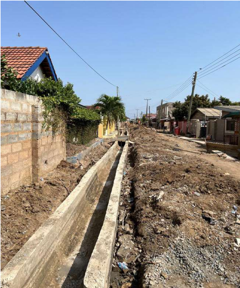
CONSTRUCTION OF U-DRAINS WITHIN THE MUNICIPALITY
