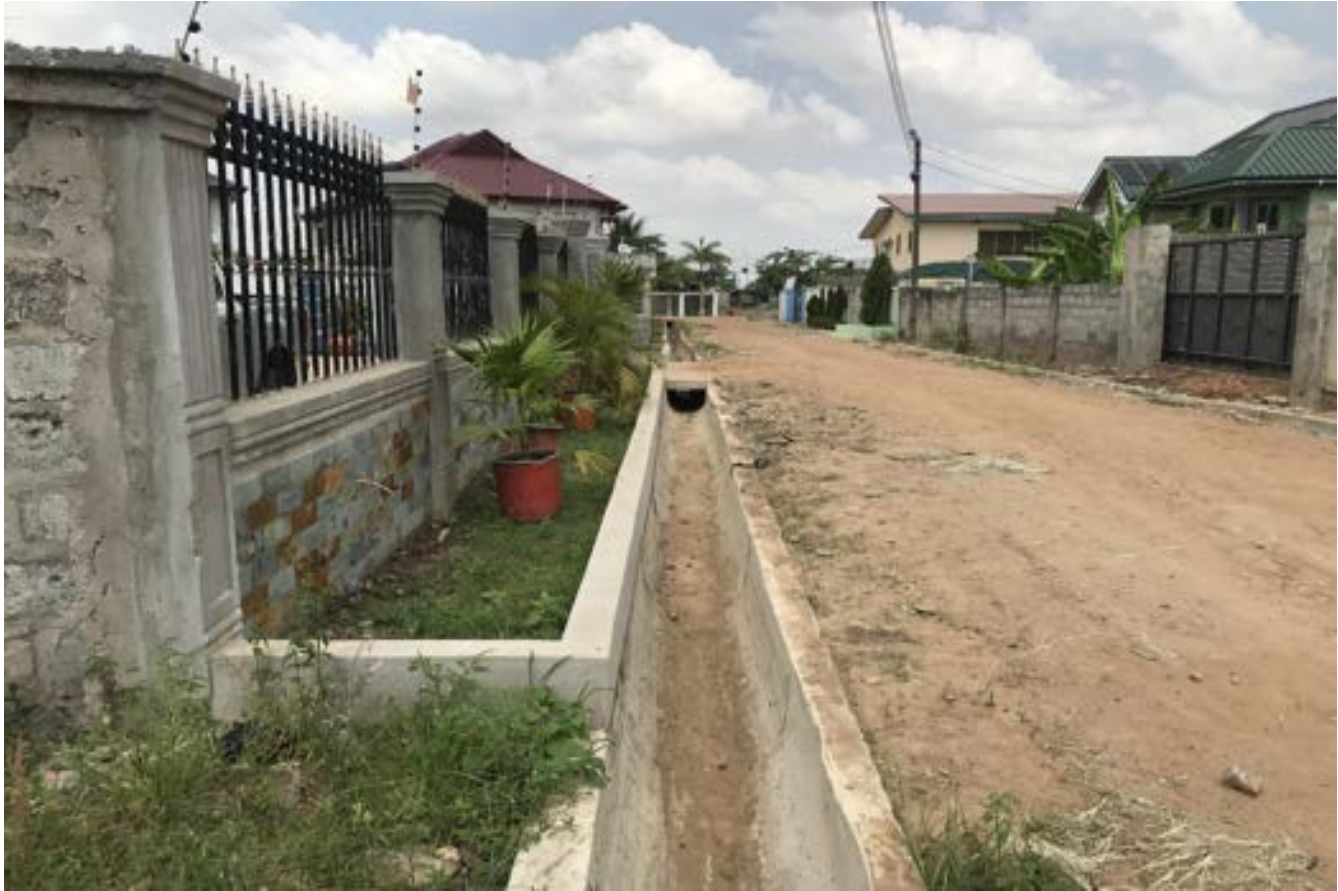
DRAINAGE WORKS ALONG KOJO MENSAH LOOP IN C14 ANNEX LOT -2
