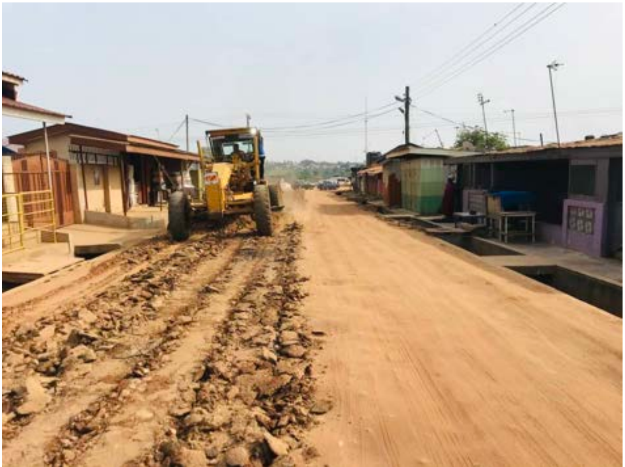
PICTURES OF GRADING ROAD WORKS WITHIN THE MUNICIPALITY
