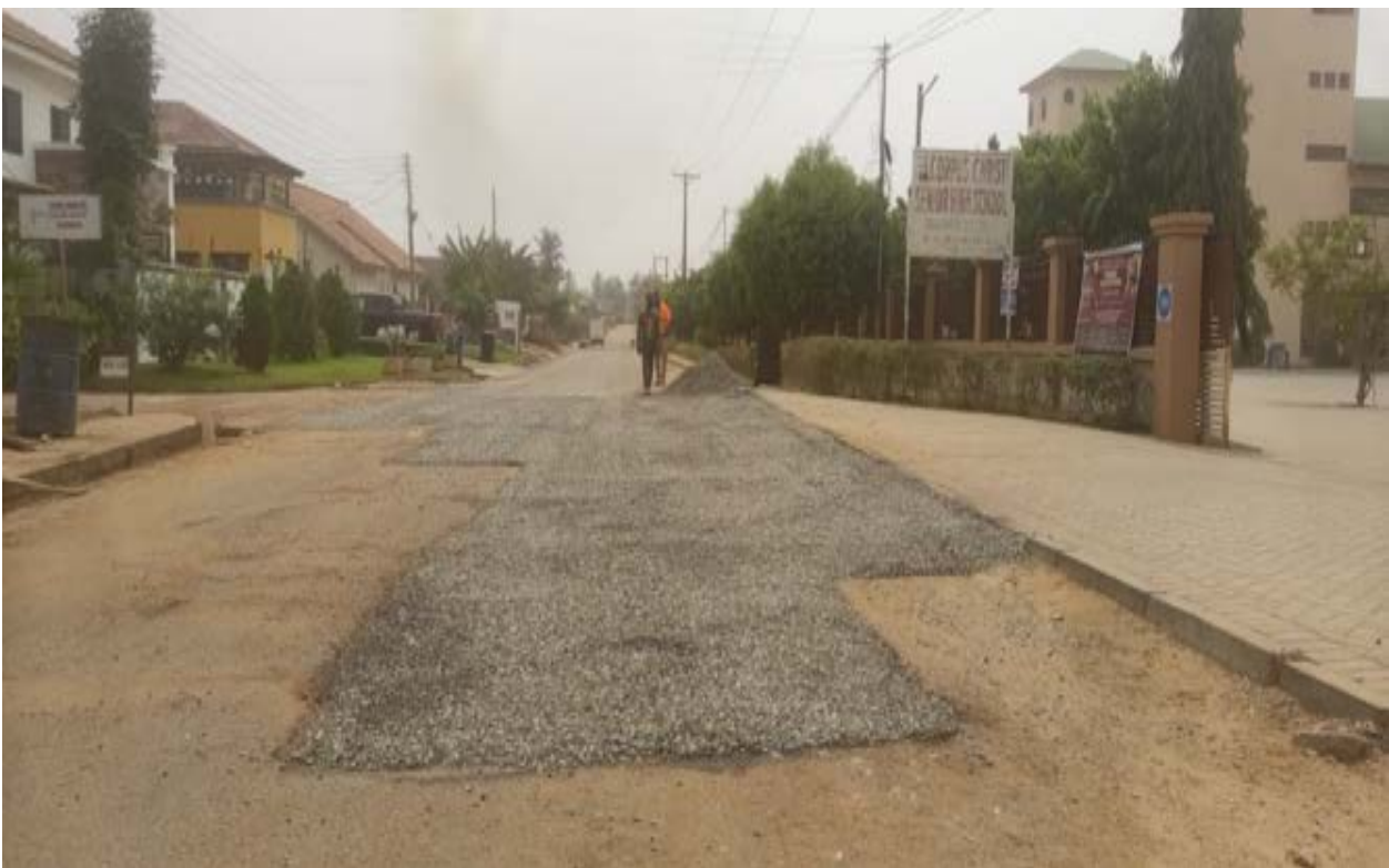
POTHOLE PATCHING WORKS ON SELECTED ROADS WITHIN THE MUNICIPALITY.
