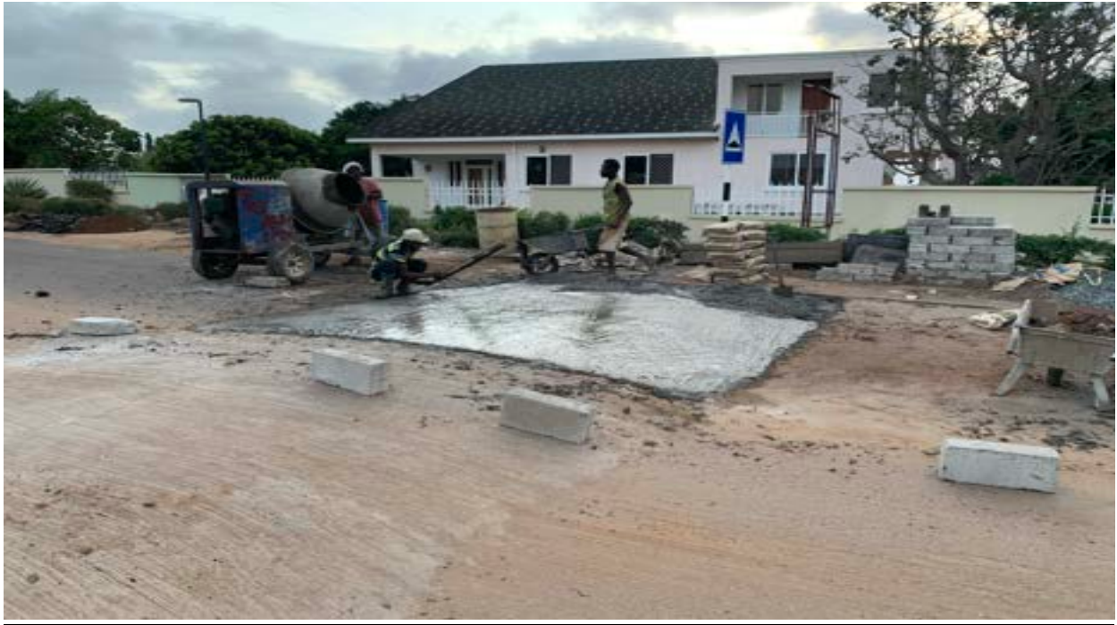
PICTURES OF CONSTRUCTION OF SPEED HUMPS WITHIN THE
