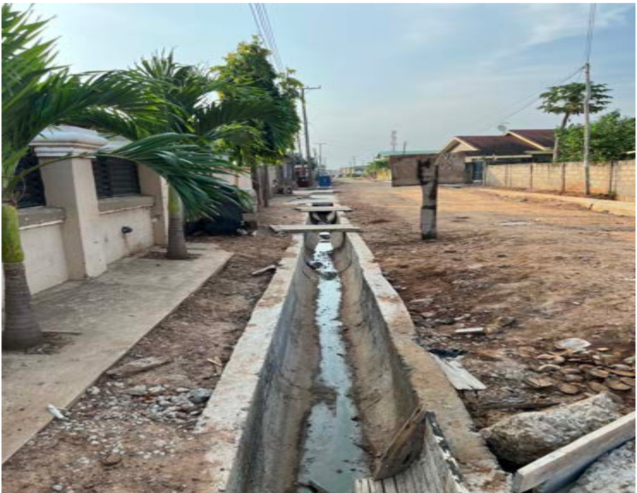
PICTURES OF DRAINAGE WORKS AT KLAGON WITHIN THE MUNICIPALITY
