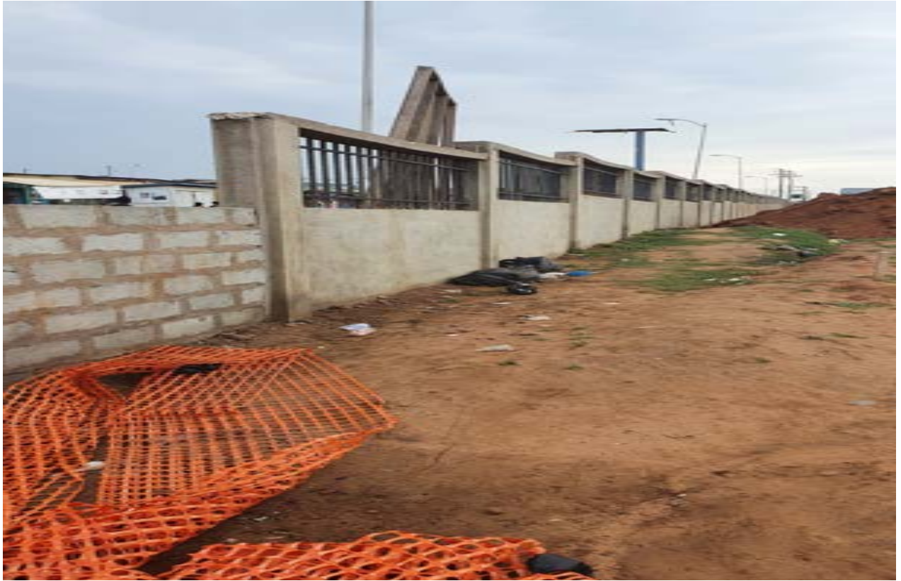
CONSTRUCTION OF SANDCRETE BLOCK FENCE WALL AT SAKUMONO TWMA BASIC SCHOOL (DACF)
