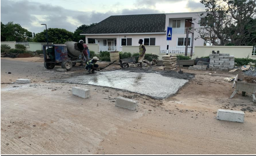
PICTURES OF CONSTRUCTION OF SPEED HUMPS WITHIN THE MUNICIPALITY
