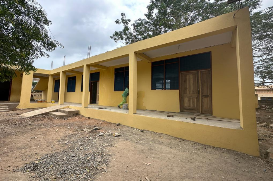
CONSTRUCTION OF 6-UNIT CLASSROOM BLOCK AT STAR BASIC SCHOOL COMMUNITY 5
