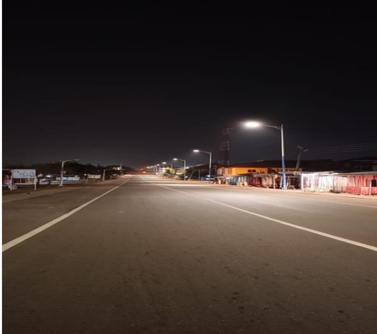
PROCUREMENT, REPLACEMENT AND REPAIRS OF STREETLIGHT WITHIN THE MUNICIPALITY
