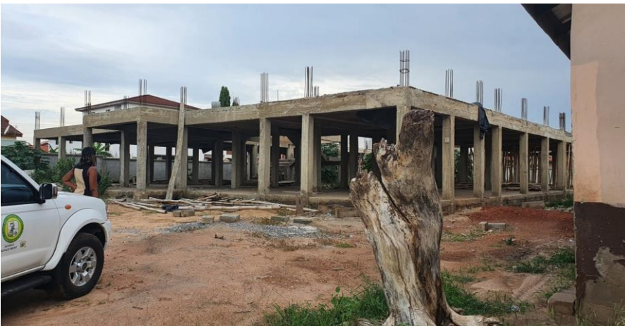
CONSTRUCTION OF 2-STOREY 12-UNIT CLASSROOM BLOCK AT LASHIBI (DACF)
