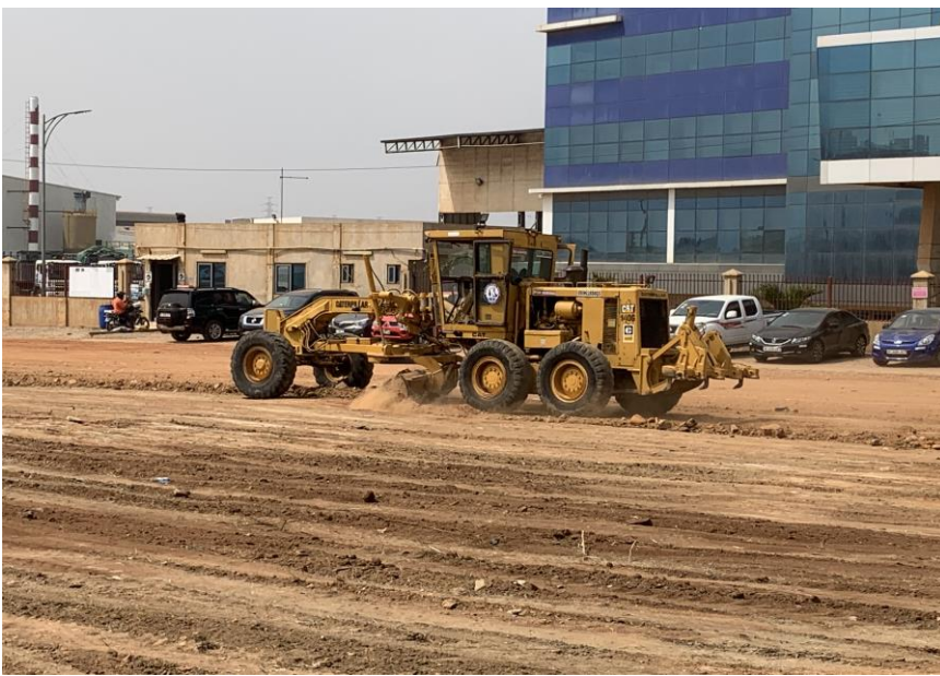
PICTURES OF SURFACING AND GRADING ROAD WORKS IN THE MUNICIPALITY
