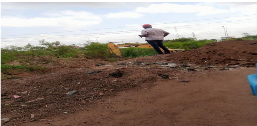
Dredging around the Akwaba oil Enclave
