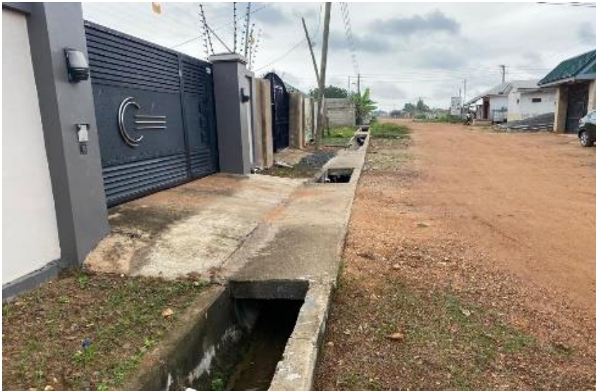
PICTURES OF DRAINAGE AND CULVERT WORKS AT KLAGON
