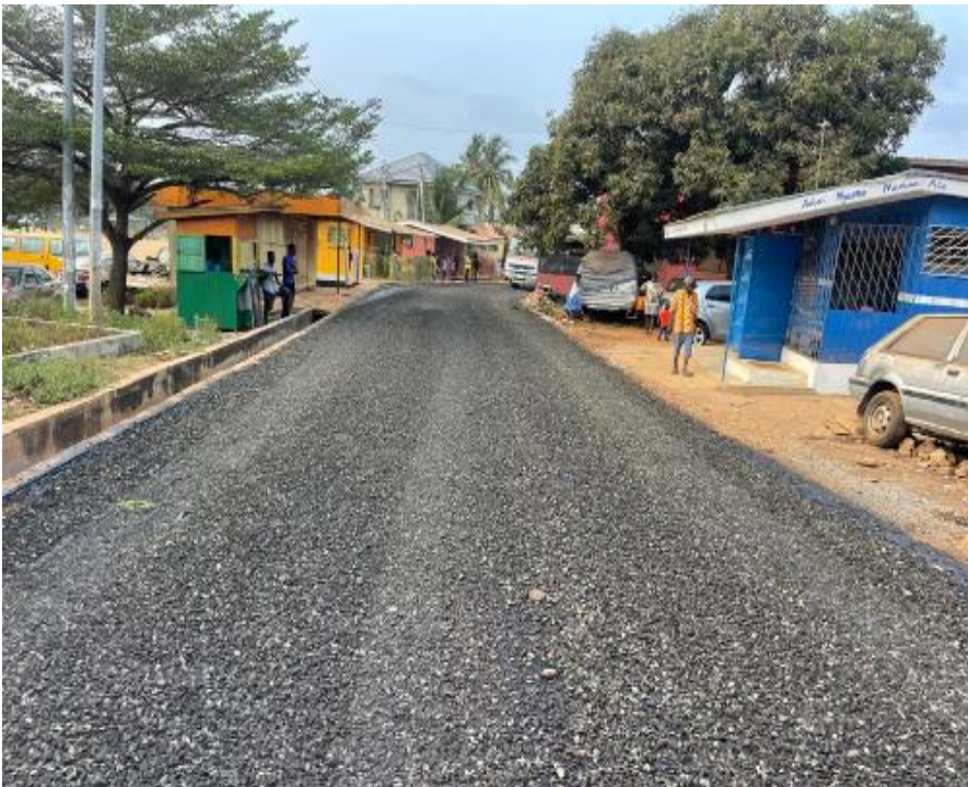
SURFACING OF ROAD AND DRAINAGE WORKS AT BORLA PITO, COMM 2
