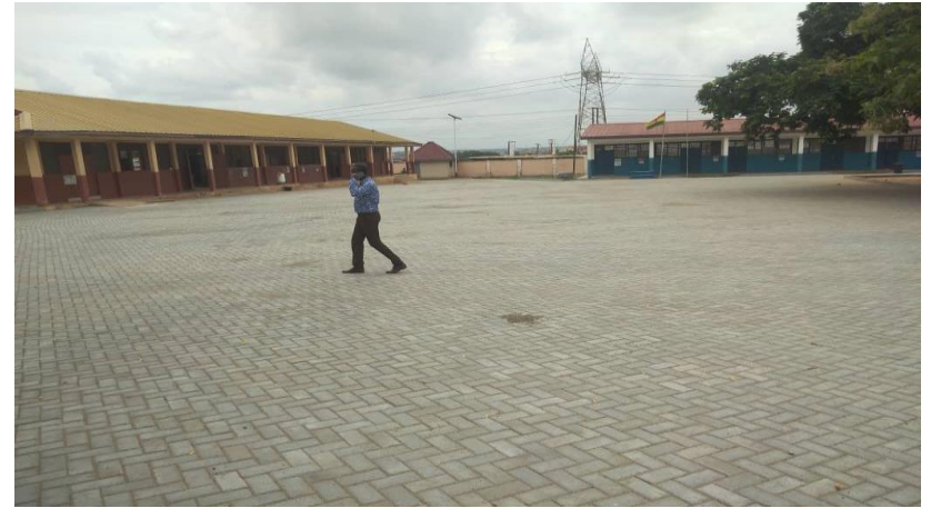
CONSTRUCTED PAVEMENT OF COMPOUND AT TETTEH OCLOO SCHOOL FOR THE DEAF, ADJEI – KOJO
