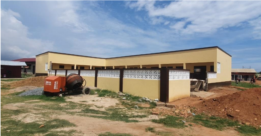
CONSTRUCTED 4-UNIT KG BLOCK AT ADJEI KOJO BASIC SCHOOL COMPLEX
