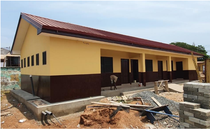
CONSTRUCTED A 3-UNIT CLASSROOM BLOCK AT MANKOASE DAY CARE CENTRE COMMUNITY 2
