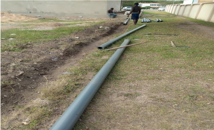
REPLACEMENT OF SEWER PIPES
