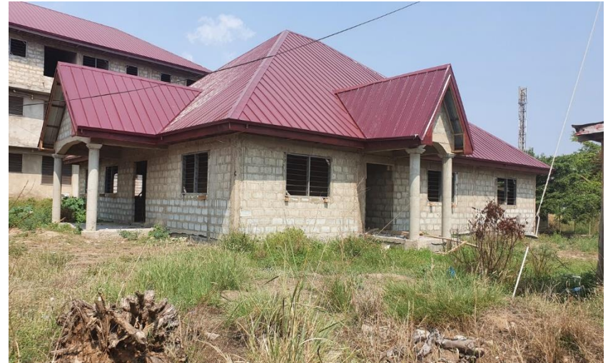
CONSTRUCTION OF COMMUNITY LIBRARY AT COMMUNITY 14 (ON-GOING)
