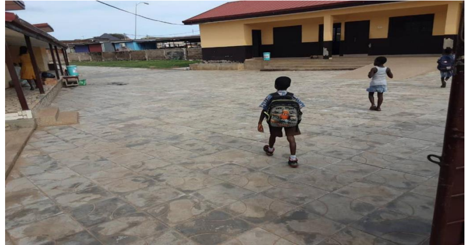
FURNISHING, LANDSCAPING AND PAVEMENT OF MANGOASE DAY CARE SCHOOL (DACF)
