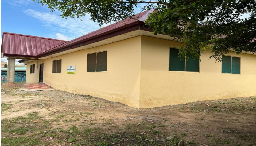
CONSTRUCTION OF A LIBRARY AT SAKUMONO (DACF)
