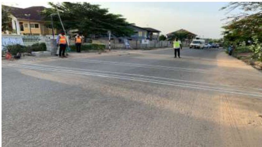
CONSTRUCTED SPEED HUMPS ON EZRA ROAD
