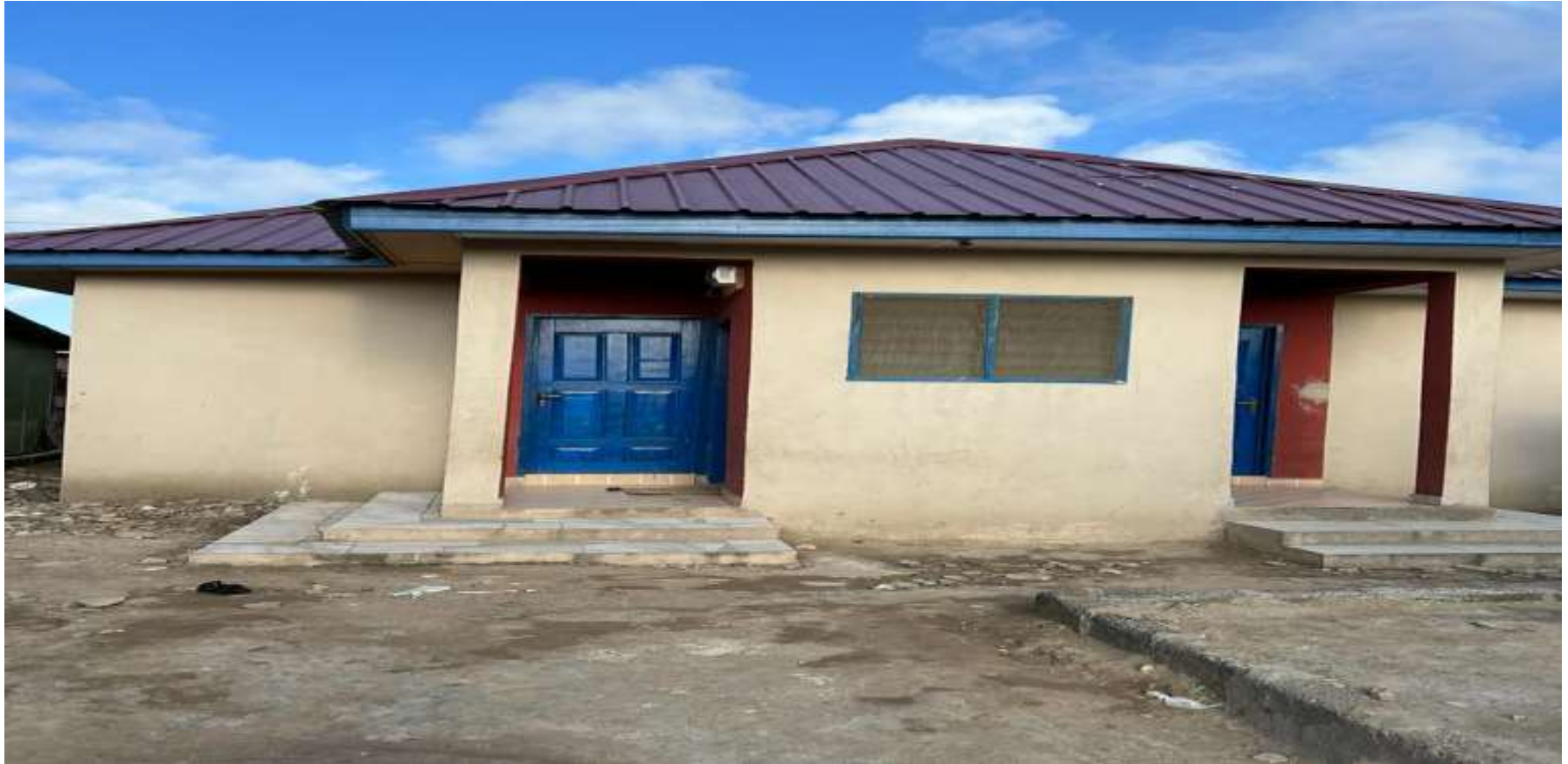
Constructed 10-Seater Toilet Facility at Texpo Market.
