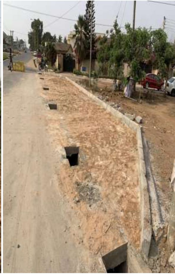
AWAITING METAL GRATINGS
