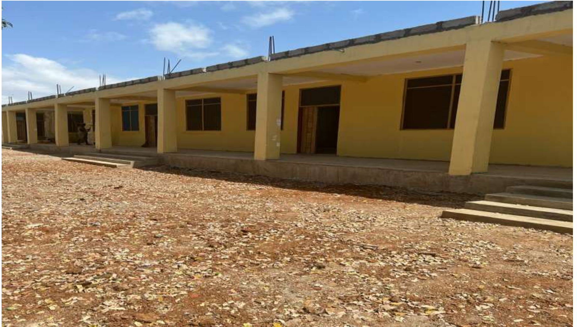
Constructed 3-Unit Classroom Block Extension at Star Basic School (Phase 1 & 2)
