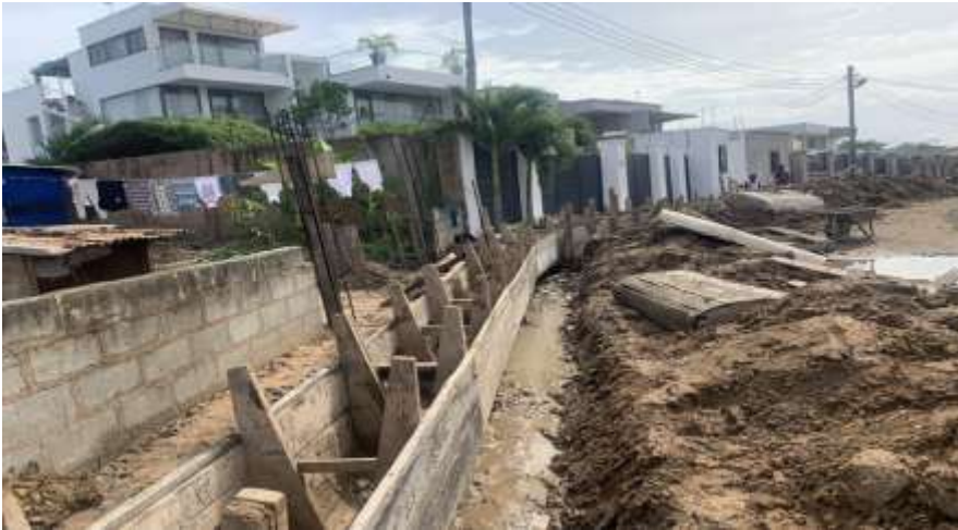
CONSTRUCTED U-DRAINS ALONG TENSIL TOWN, KOJO MENSAN LOOP
