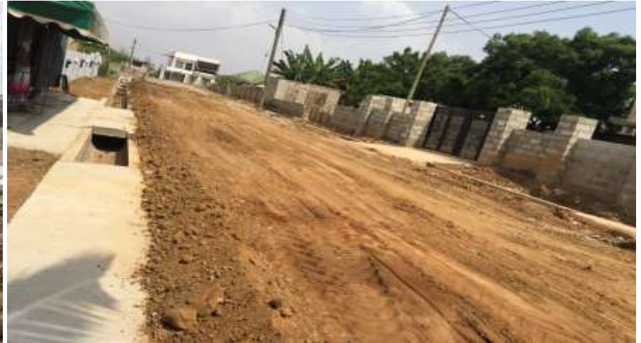
CONSTRUCTED U-DRAINS ALONG TENSIL TOWN, KOJO MENSAN LOOP
