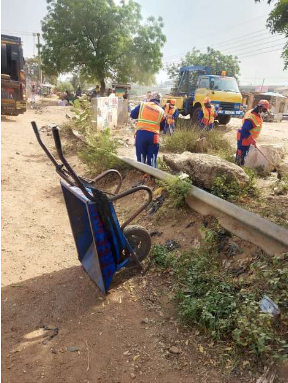
CLEANUP EXERCISE UNDERTAKEN ALONG THE MOTORWAY
